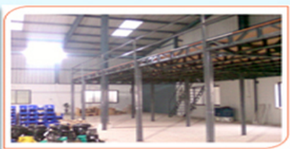
Mezzanine Floor With M.S. Slotted Angles
